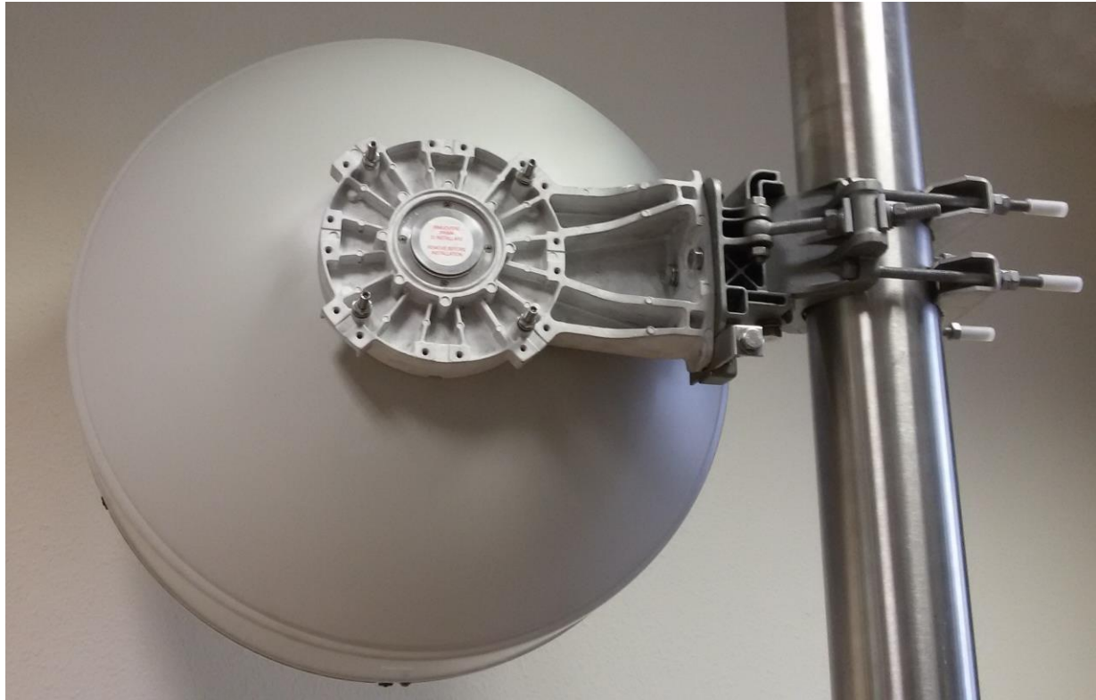
Figure 3.1-6: Integrated antenna1+0 mounting
