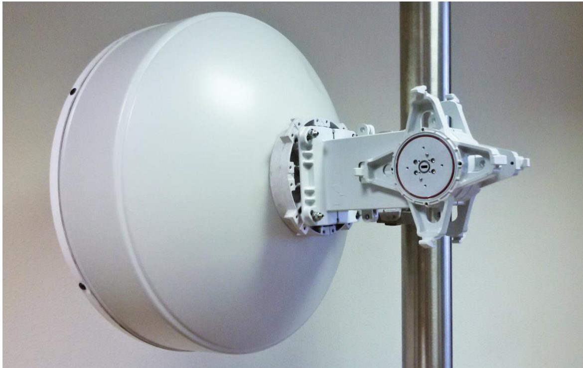
Figure 3.1-8: Integrated antenna1+1 / XPIC mounting
